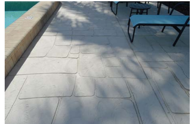
POOL DECK / PATIO
