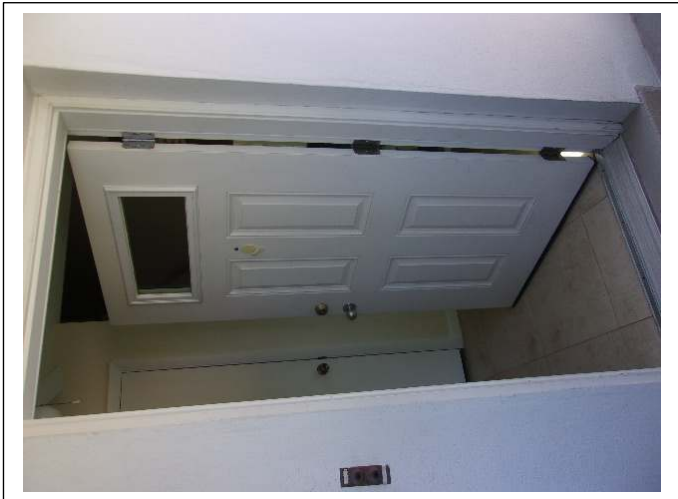
OPENING PROTECTION – The glazed front entry door is large missile rated. FBC# FL17184.21
