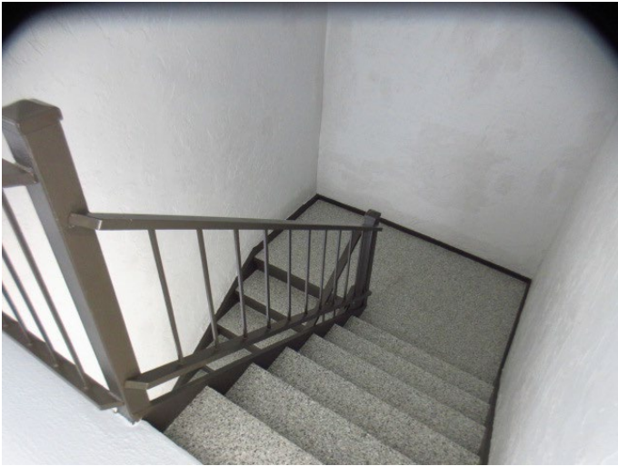
VIEW OF STAIRS
