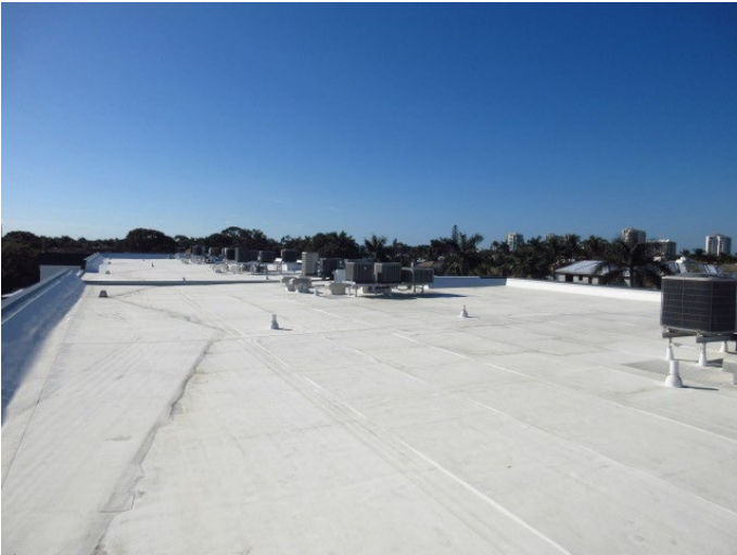
GENERAL VIEW OF ROOF COVERING
