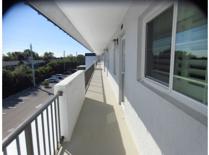
VIEW OF ELEVATED WALKWAY
