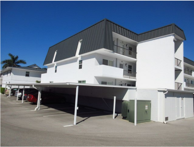
VIEW OF MANSARD ROOF
