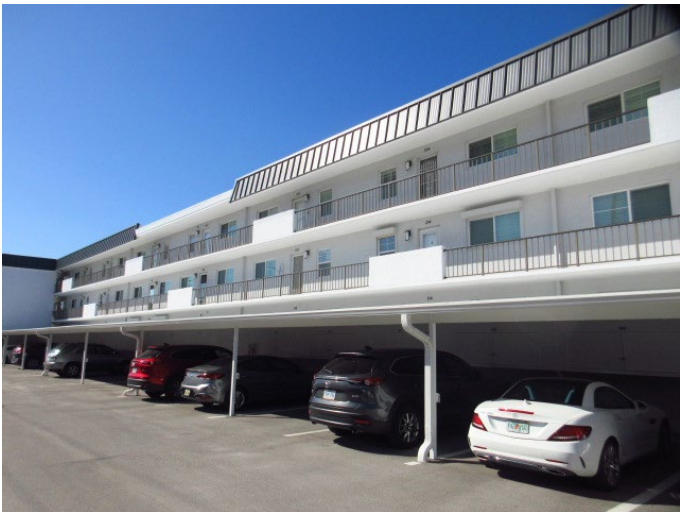
GENERAL VIEW OF BUILDING EXTERIOR FINISHES
