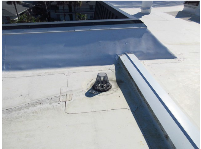
GENERAL VIEW OF ROOF DRAIN
