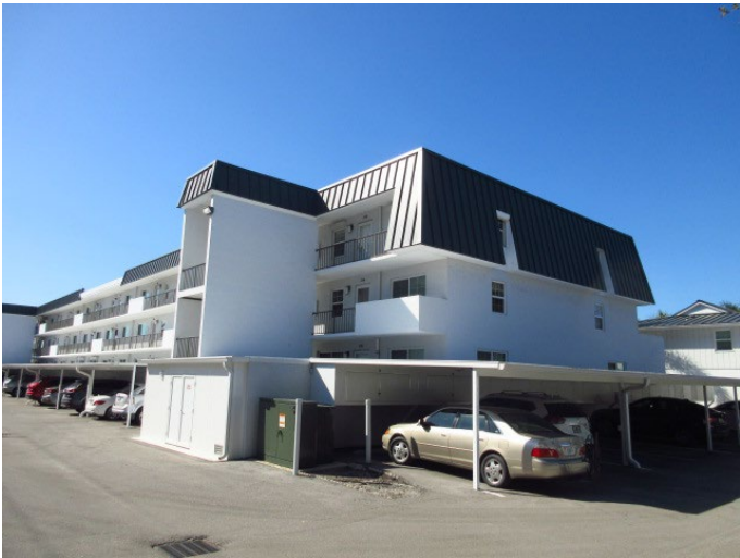
VIEW OF BUILDING EXTERIOR FINISHES
