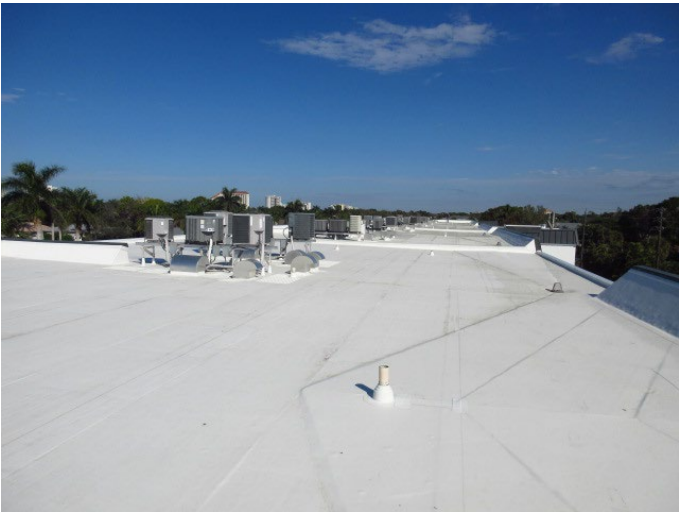
GENERAL VIEW OF ROOF COVERING
