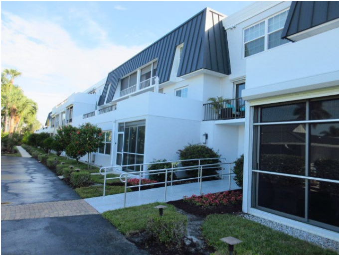
GENERAL VIEW OF BUILDING EXTERIOR FINISHES
